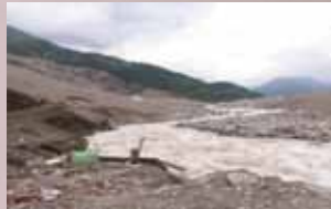
Draining of overflow from dam
